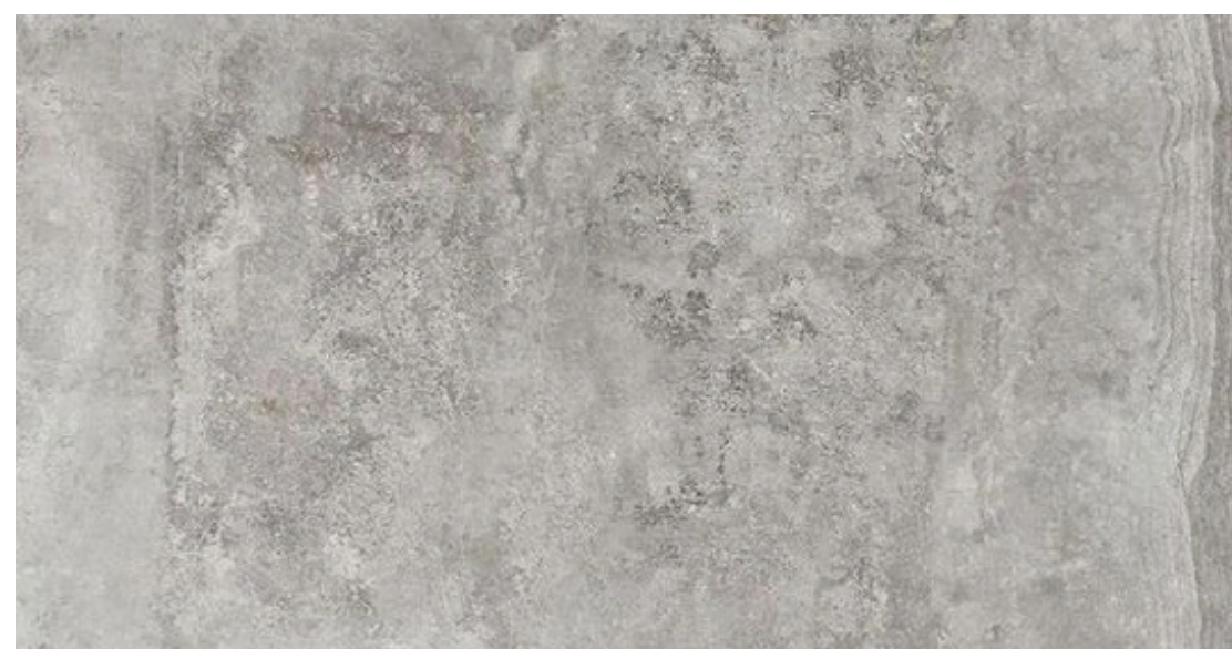
Ceilings Concrete ceilings
